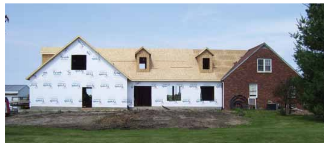
Former rental house with new addition
