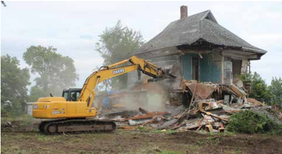
Demolition and clean up in progress.
