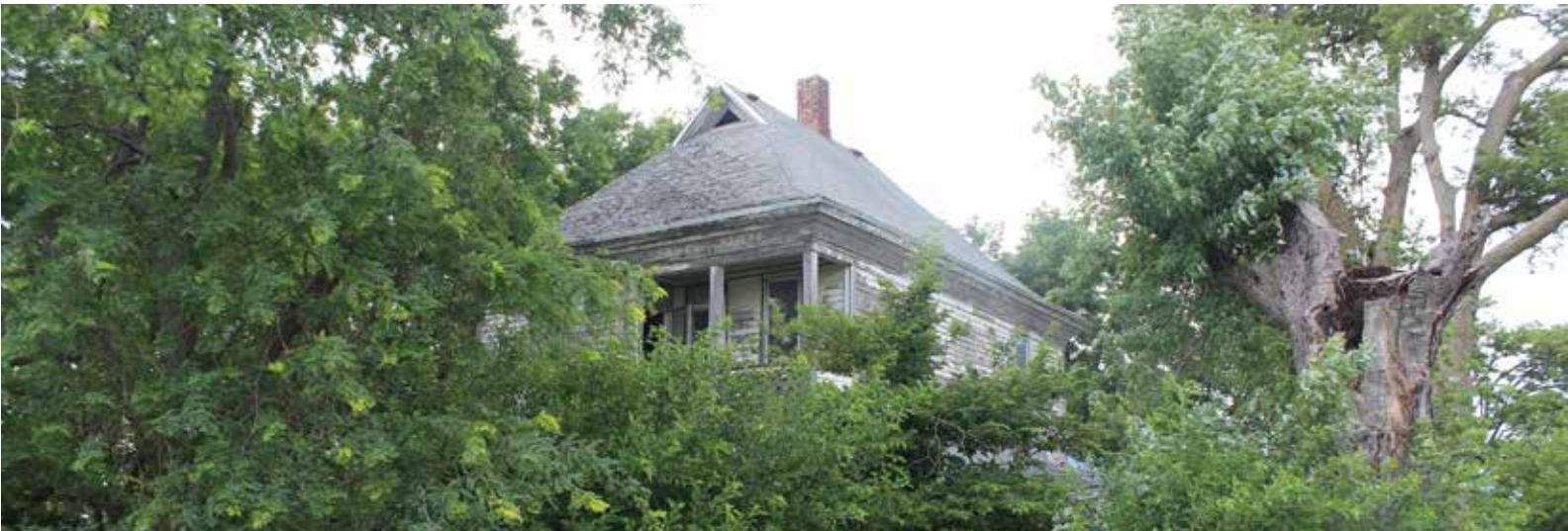
Farm property prior to demolition and clean up.
