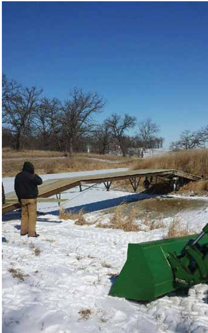
Setting the bridge in place.
