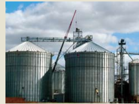
Maintenance work on grain system.
